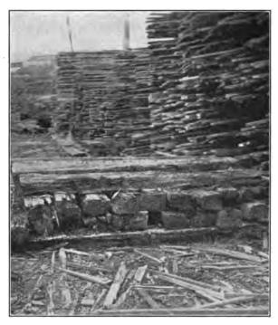
Fig. 86.—A highly insanitary mill yard in South Carolina. Hundreds of thousands of feet of stored lumber have rotted in this yard as a result of these conditions. All this rotten débris should be removed and burned.
